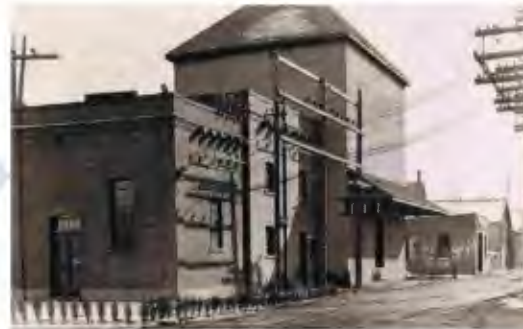
Collingwood's 1952 sub-station housing—six 667-KVA transformers were erected on St. Marie Street
