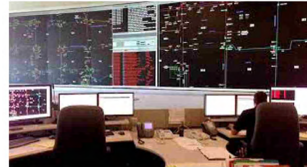
PowerStream state-of-the-art Control Room
