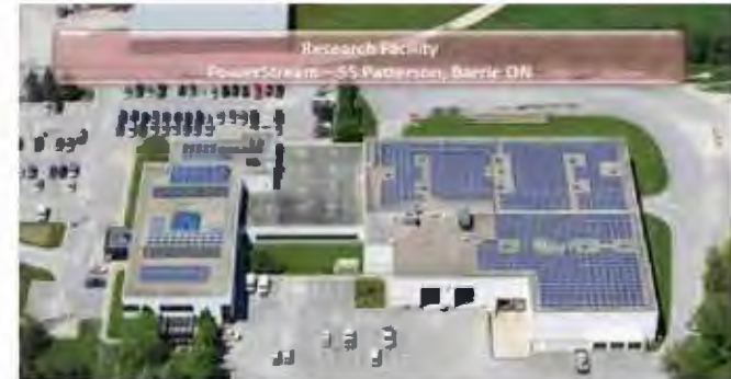
PowerStream Facility in Barrie
