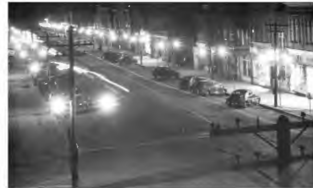
Traffic lights were installed on Hurontario Street in 1948, at the intersections First, Second, Third and Hume streets to control increasing automobile traffic.
