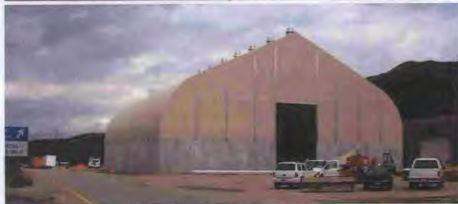
Salt/Sand Storage Facility Vail Pass, Colorado Rockies
