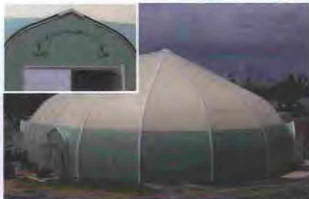
Exterior membrane replaced after Hurricane Katrina.
